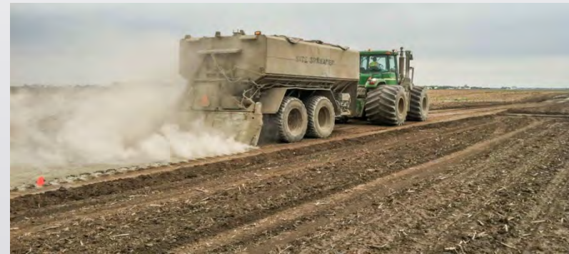
Spreading cement for soil stabilization
