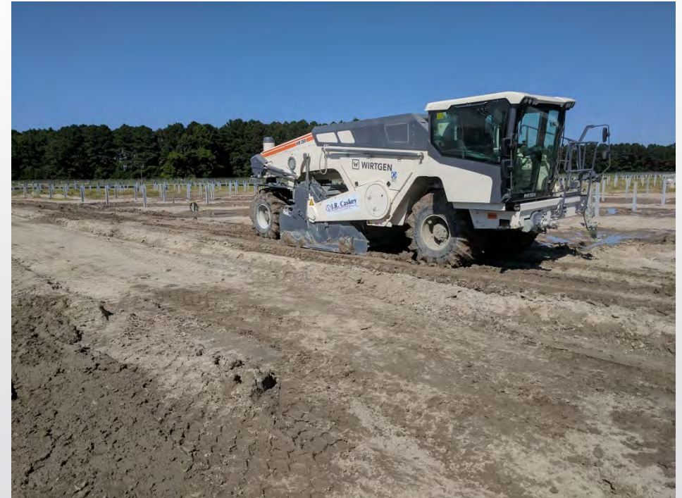
J.R. Caskey's WR-250 mixing cement to a depth of 18"
