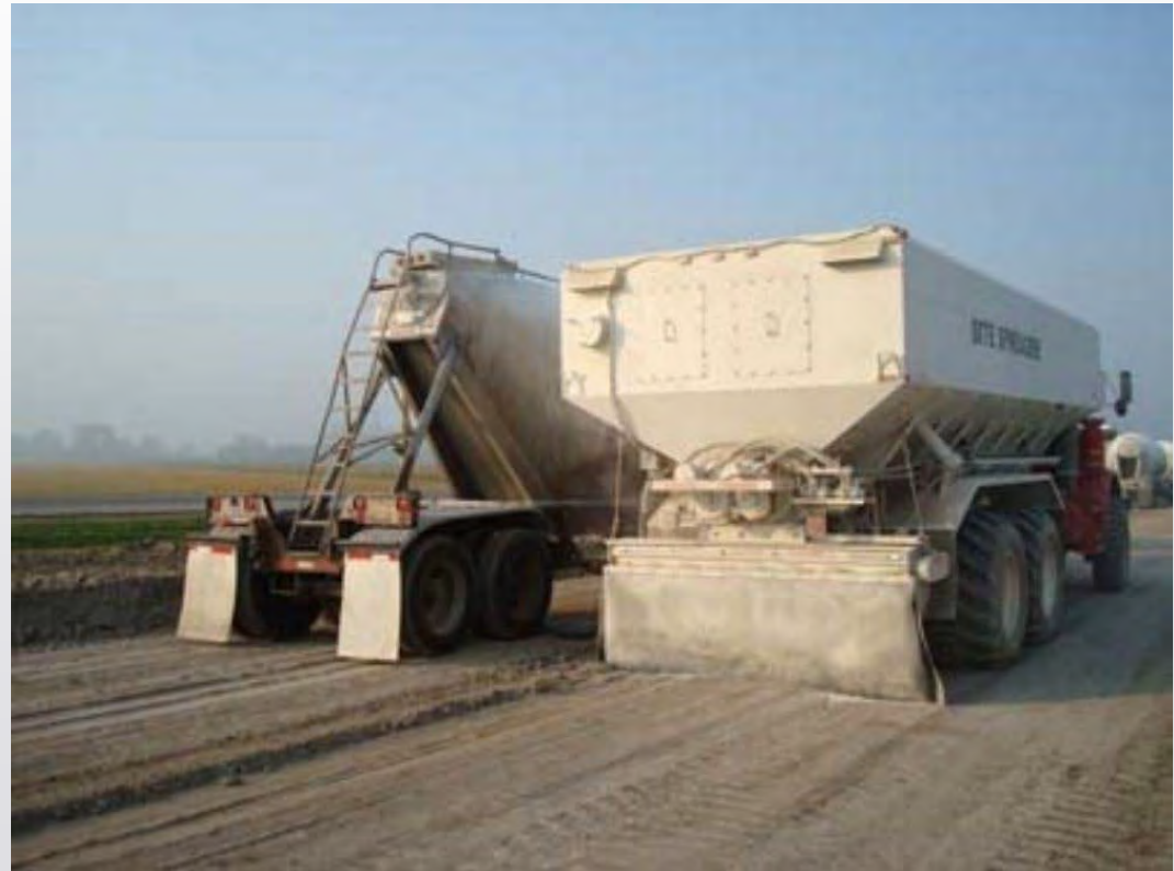
Cement tanker and spreader wagon
