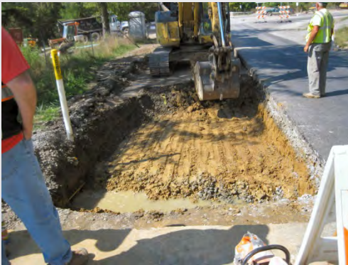
Undercut for roadway
